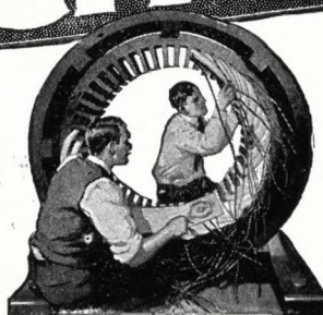
Student Winding Stator at COYNE
